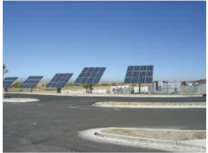
The Green Park DIA near Denver International Airport will utilize numerous strategies for energy reduction including a ground-mount solar PV system and wind turbines.
