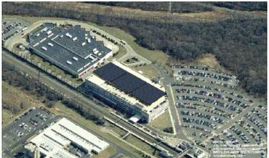
Hamilton Station park and ride with solar array installed on the roof.
