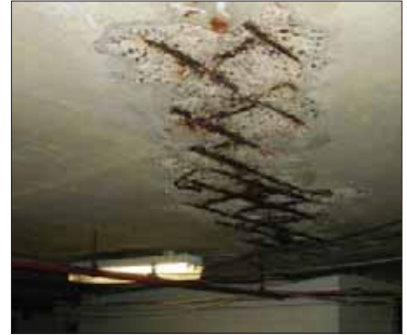
ABOVE: Structural members that show signs of deterioration such as cracking, corrosion stains, leaking water, leaching, delaminations or spalling should be reviewed by a qualified parking structure restoration engineer.
