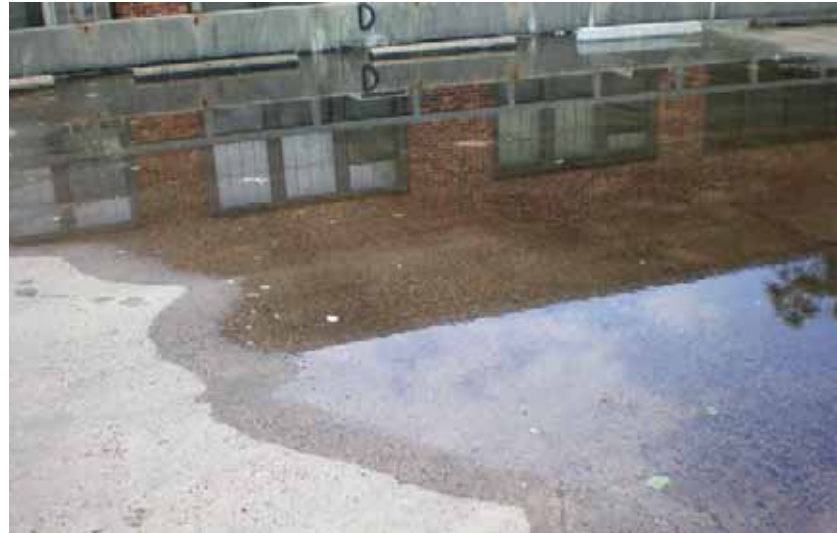
ABOVE LEFT: Leaking water from poorly maintained plumbing and fire protection systems can cause major structural damage, requiring costly repairs such as beam repair or replacement. ABOVE RIGHT: While pigeons appreciate naturally occurring bird baths, ponding water within parking structures must be corrected as it caused many issues such as accelerated structural deterioration and slip and fall hazards.
