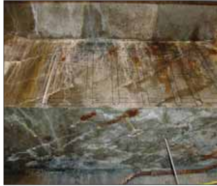
ABOVE: Structural members that show signs of deterioration such as cracking, corrosion stains, leaking water, leaching, delaminations or spalling should be reviewed by a qualified parking structure restoration engineer.
