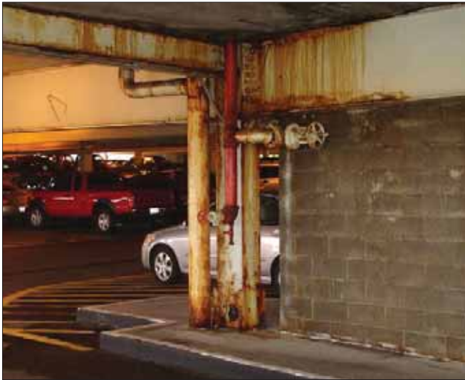
ABOVE LEFT: Leaking water from poorly maintained plumbing and fire protection systems can cause major structural damage, requiring costly repairs such as beam repair or replacement. ABOVE RIGHT: While pigeons appreciate naturally occurring bird baths, ponding water within parking structures must be corrected as it caused many issues such as accelerated structural deterioration and slip and fall hazards.
