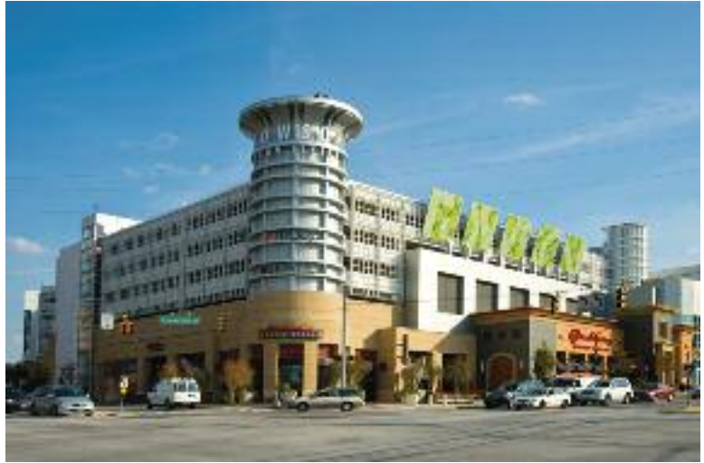
The Towson Town Center garage expansion helped to create a more vibrant “downtown” feeling, creating a more attractive pedestrian experience.
