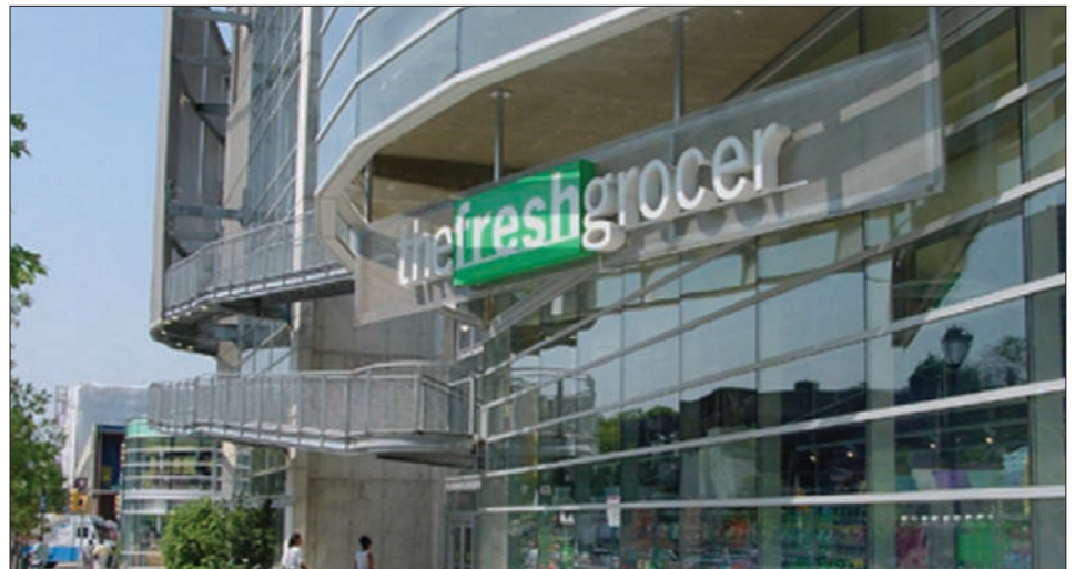
Hamilton Square: The Hamilton Square project for the University of Pennsylvania utilized the effective integration of parking and retail to create a more sustainable and attractive community to serve its students.
