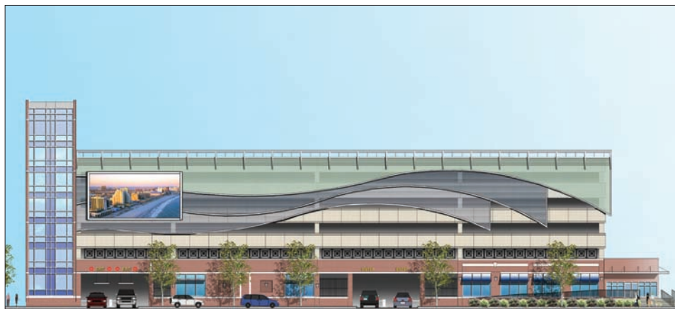
Casino Reinvestment Development Authority mixed-use parking structure in Atlantic City.
