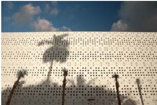
The Park@420 garage at Drexel Ave. and 16th St. in Miami Beach, designed by architect Enrique Norten.
